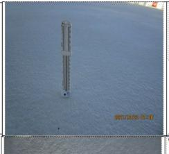
View of probe showing required 2" application of spray foam. Multiple areas were tested with the depth gauge and all were in compliance.
